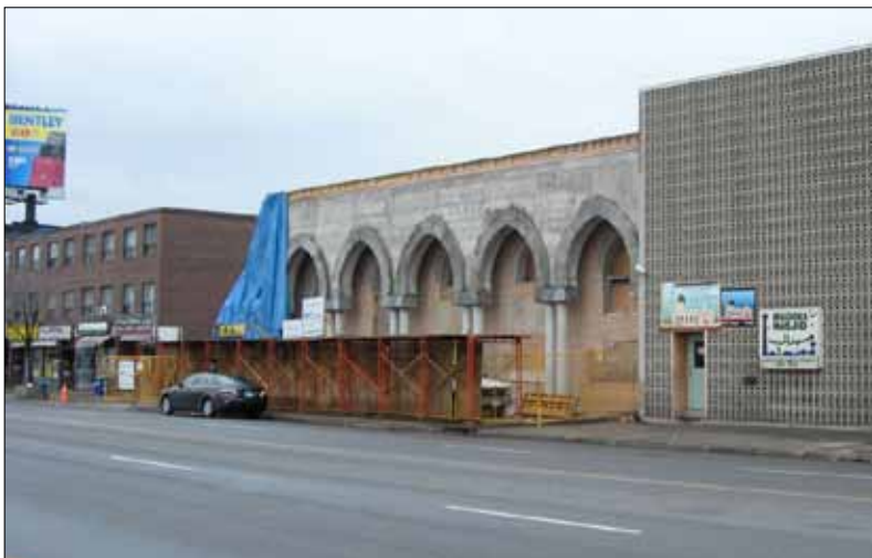
The Madinah Masjid under construction
